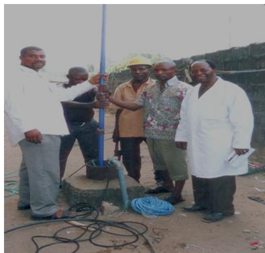
Figure 3 Shows work being done on the borehole at Awaka
